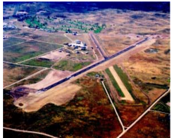
Wray Municipal Airport's new runway on the eastern plains was recently funded through the FAA's Airport Improvement Program.
